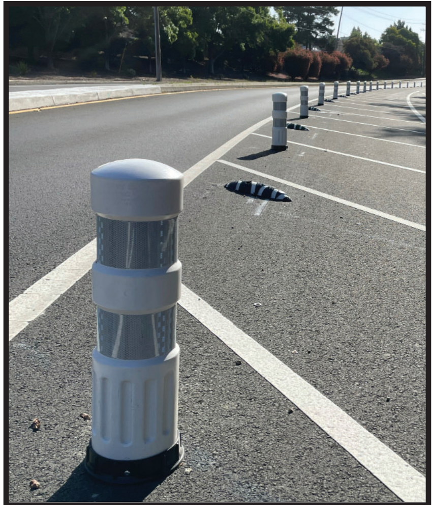
Bollard rebounds to upright position after impacts.
